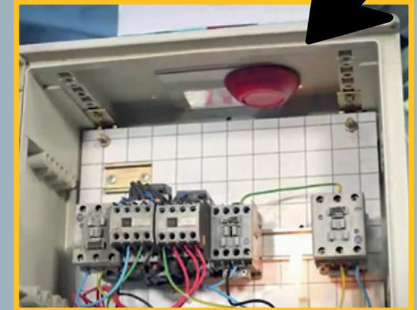
**Savio Stick Protect** is an automatic thermal aerosol device developed as an aid in extinguishing fires caused by short circuits. It is particularly suitable for domestic, industrial, and marine applications.
